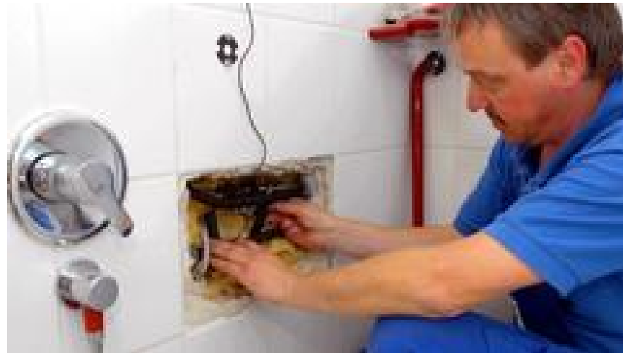
Klaus-Dieter Paul has installed a regulator in «Rainbow», with its help legionella bacteria should be prevented.
